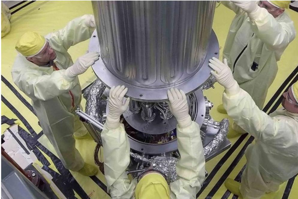
\*NASA and National Nuclear Security Administration engineers lower the wall of a vacuum chamber around the Kilo power reactor system
