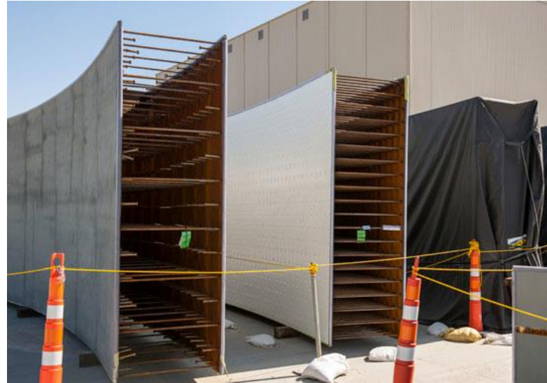
Vogtle Unit 3 shield building wall panels, May 2014
