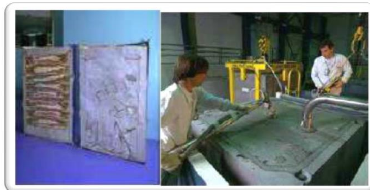
Stabilization by solidification of nuclear waste
