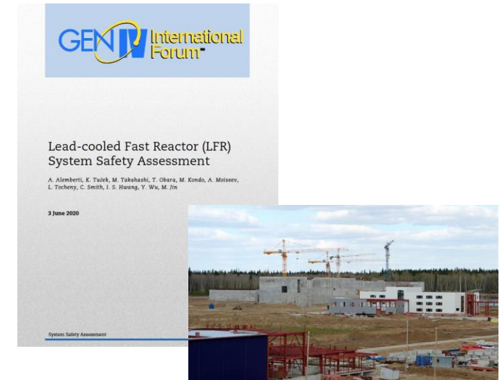
Site preparations for the BREST-OD-300 construction
