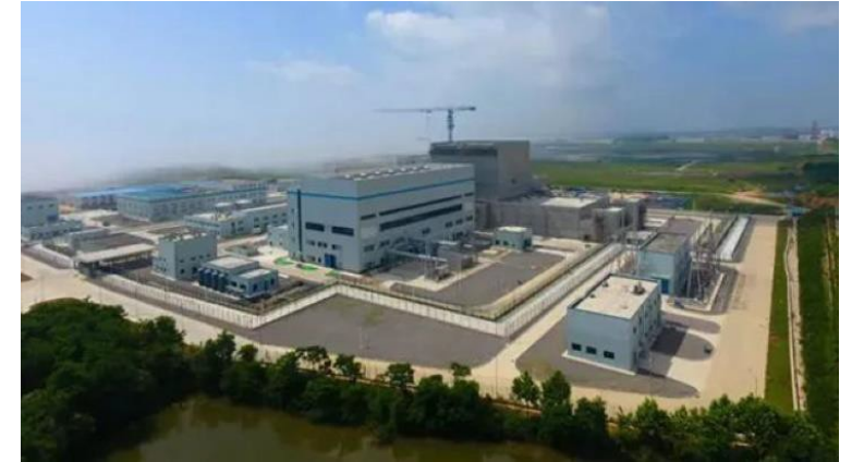
Construction site of HTR-PM
